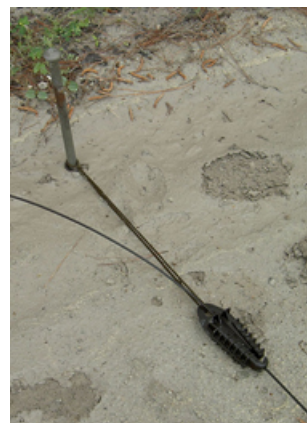
Wedge clamp in operation
